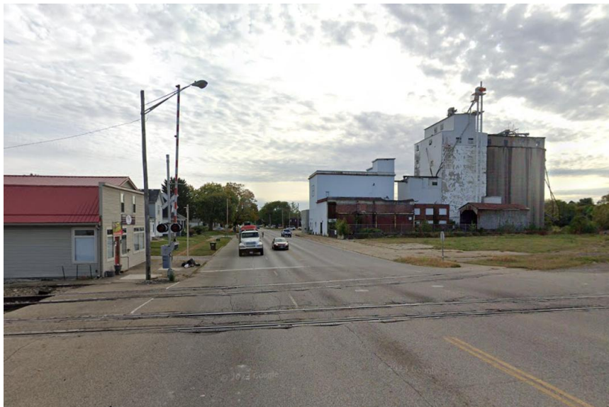
Existing at-grade railroad crossing at S Court Street, looking south.
