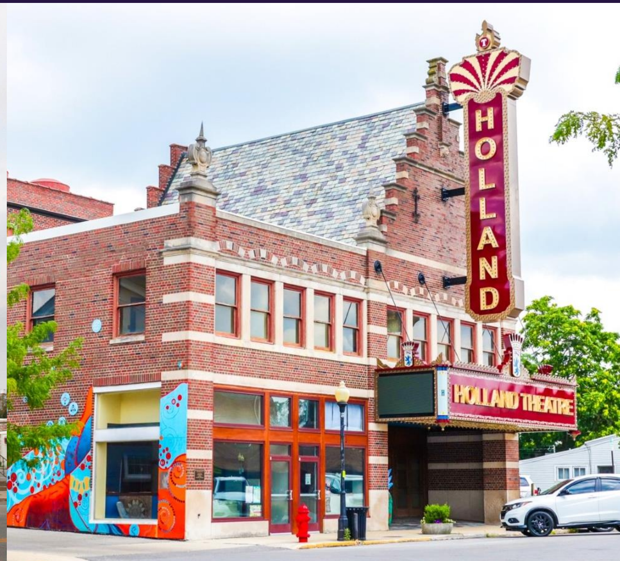
Holland Theatre Before and After with Jeffris Grant
